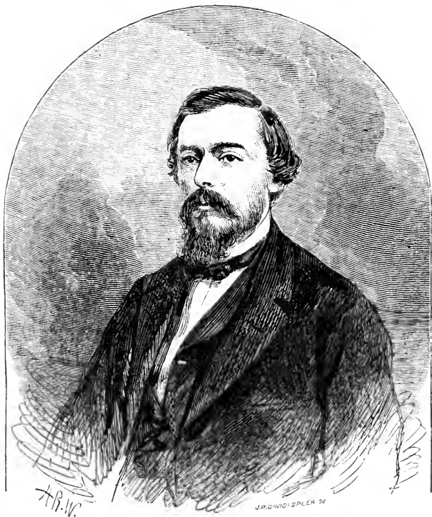
THOMAS C. DURANT, BUILDER OF UNION PACIFIC RAILROAD.
